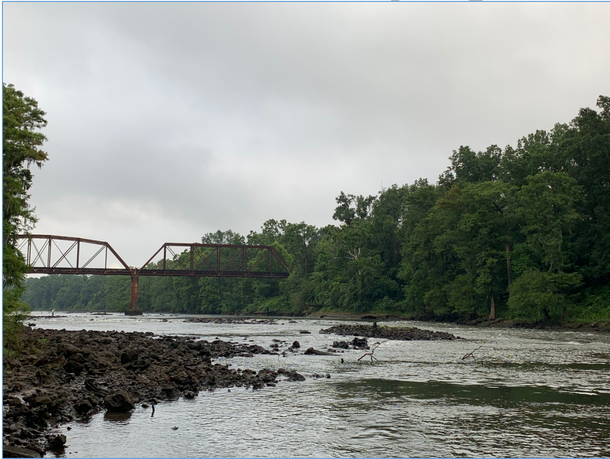
Figure 5: Limestone outcrop along the Flint in downtown Albany.
